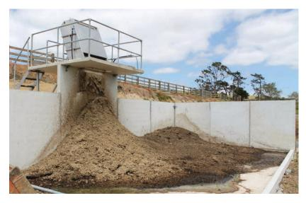
Typical static screen and bunker installation
