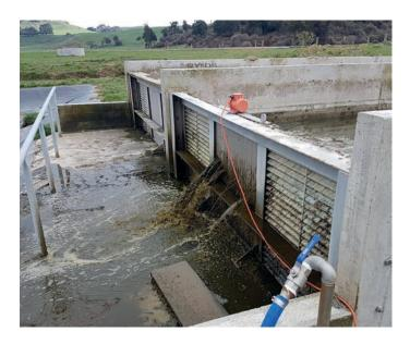
Weeping wall (PVC outer panels, vibrating centre panel)
