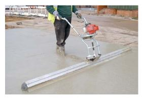
Figure 11: Lightweight vibrating screed
