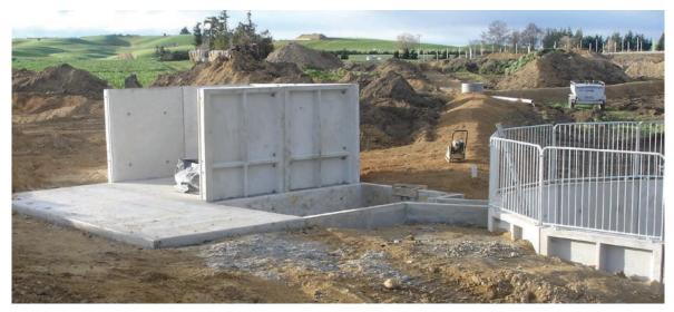
Reinforced concrete storage bunker with draining pad, stone-trap and sump
