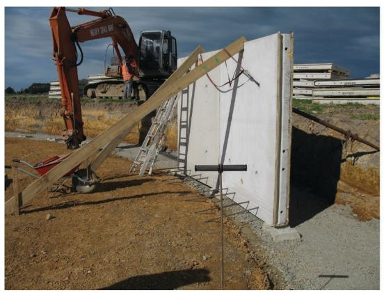
Storage tank, precast reinforced concrete panel construction
