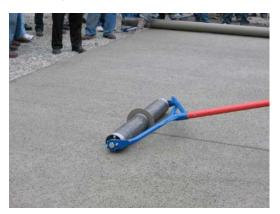
Figure 18: Jointing tool or T section
