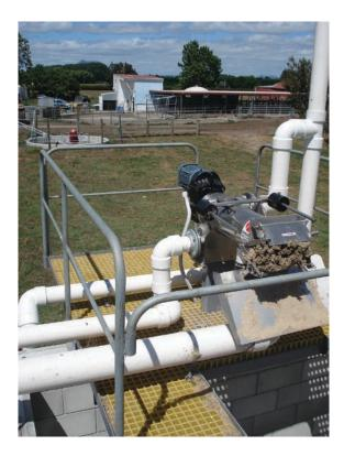
Typical screw press installation
