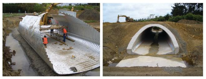
Galvanised steel corrugated multiplate culvert underpass under construction
