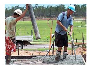
Figure 12: Immersion poker vibration
